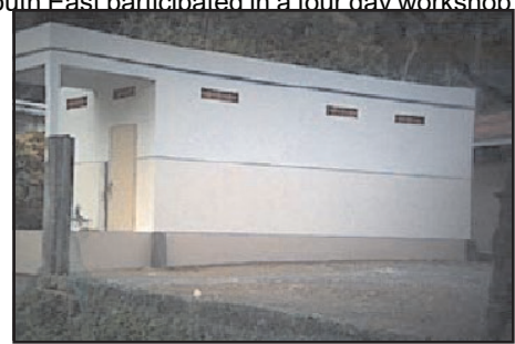
Castries South East Satellite Warehouse
